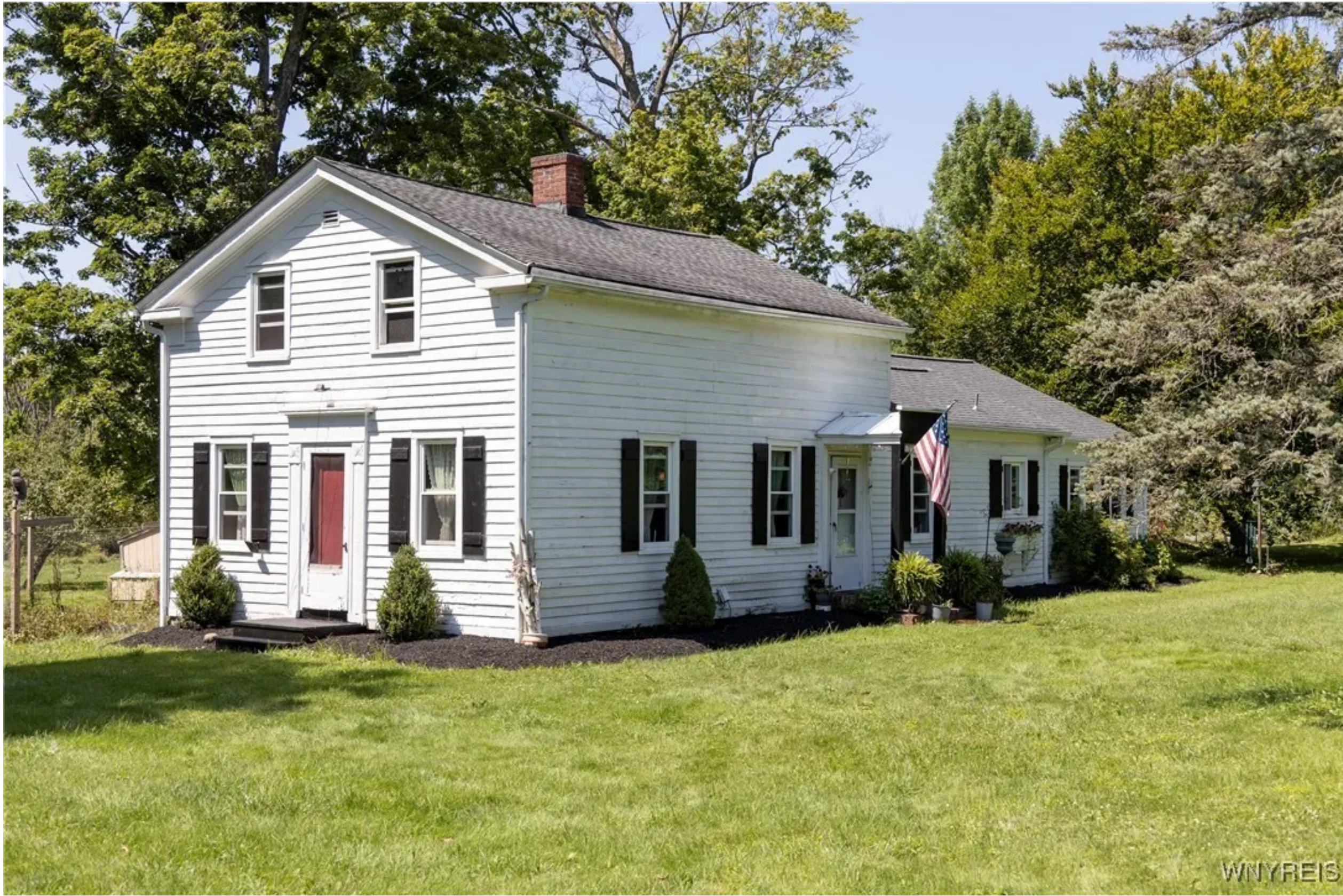
EXISTING SLEEPING QUARTERS
