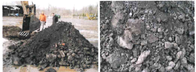
Mostly rocky slag fill spoils, with cemented layers, unable to penetrate bottom layer. Noticeable odor, 250 ppm PID reading from spoils.
