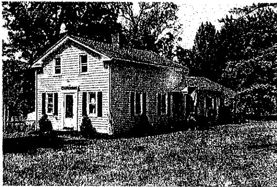
EXISTING SLEEPING QUARTERS
